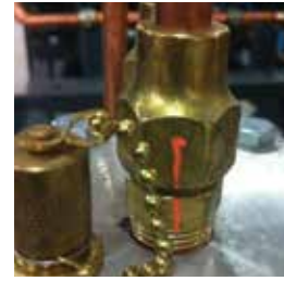
A torqued mechanical connection.
