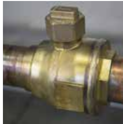
A torqued electrical connection.
