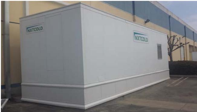
NXTCOLD's ultra-low ammonia charge of 6 to 8 oz. per ton is the lowest charge ammonia refrigeration solution available for large refrigeration facilities. As a result, it is not subject to the same extensive regulatory mandates as large ammonia charge systems. The units are delivered preassembled after undergoing rigorous quality control inspections at Hillphoenix. This attention to every detail results in less complicated installation and startup than traditional industrial systems.
