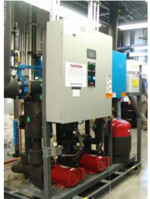
Conventional SNMT system with constant-speed (CS) pumps
