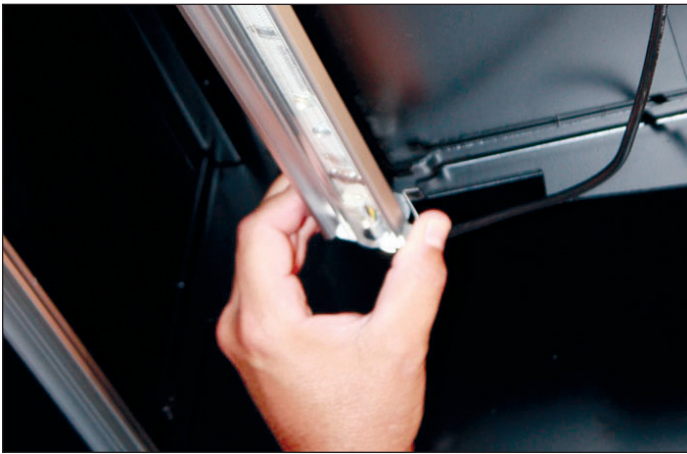
Fig. 11 Remove the old LED luminaire
