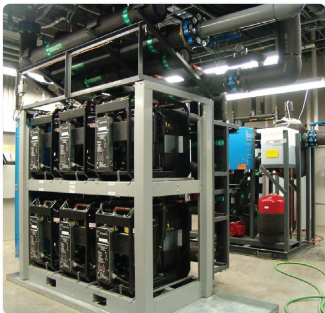
A compact chiller module (CCM) rack and a fluid pump station.
