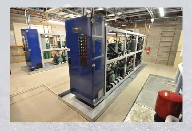
The Hillphoenix $^*$  Advansor  $\mathrm{CO}_2$  booster system is a member of our sustainable line of refrigeration systems. The Advansor  $\mathrm{CO}_2$  booster system is an HFC-free refrigeration alternative that utilizes carbon dioxide as the only refrigerant in the system. Hillphoenix customers can take advantage of the inherent benefits of  $\mathrm{CO}_2$  and combine them with those of other Second Nature systems - reducing direct refrigerant emissions to the lowest level possible.
