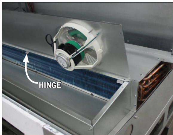
Fig. 15 Pressure plate and hinges (underside)
