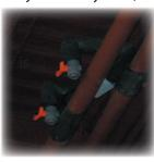
i. Vent air from the system starting at the lowest vent points and moving continually to higher vent points until all air purged from system including main vent lines again
