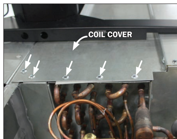
Fig. 15 Coil cover removal
