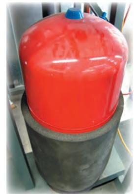
4. Verify that the pre-charge pressure in the expansion tank is at 12 psig
