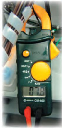
e. If amperage is too high, reduce by closing pump outlet balance valve until the proper amperage is reached
