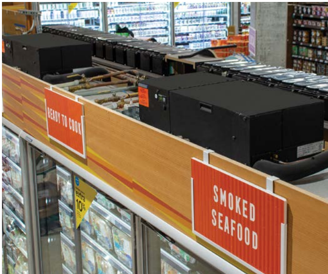
SoloChill — A micro-distributed system in a small, compact design with a smaller charge (<50 Lbs) of lower GWP synthetic refrigerant.
