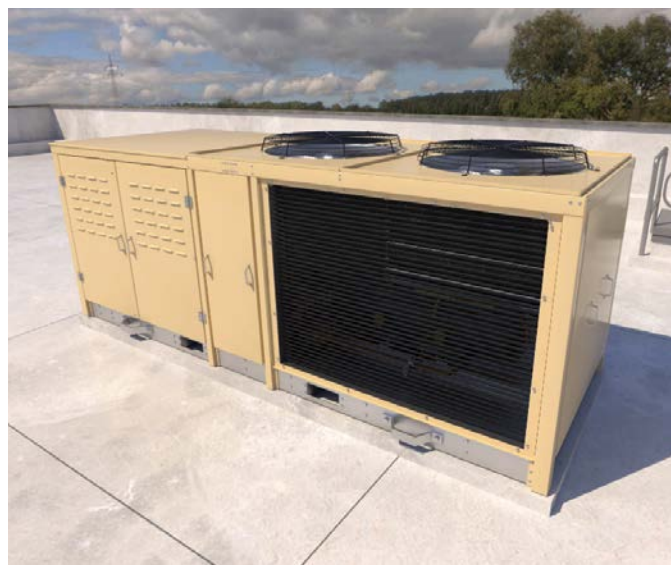
Adaptapak — utilizing a lower GWP, synthetic refrigerant, these distributed systems are mounted outside with a low-profile, compact design that is less noticeable.
