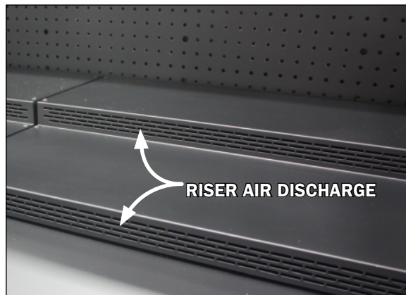
Fig. 21 Step riser perforated front air discharge
