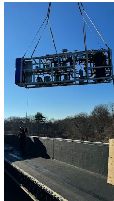
Figure 5: Lowering rack through roof
