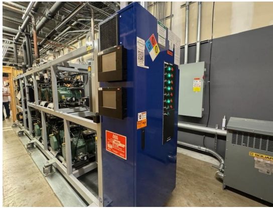
Figure 6: Hillphoenix Advansor CO 2 system
